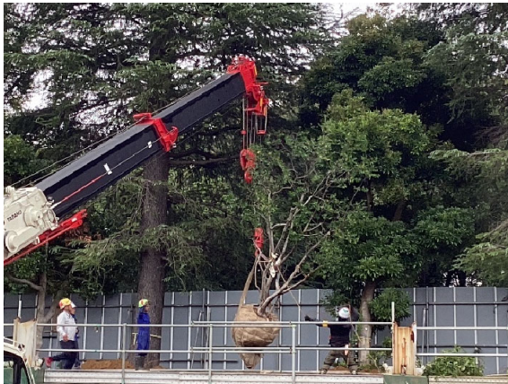
Hoisting carefully protected tree out of the ground for transplantation
